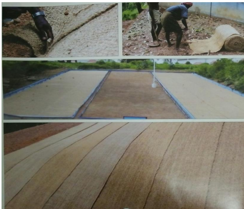
Laying of coir geotextile
