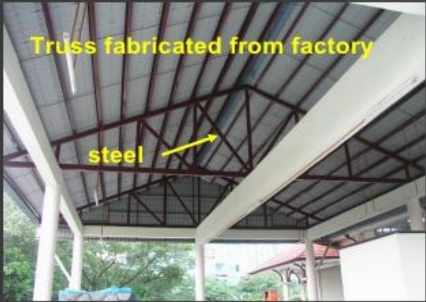
Whole roof structure built from steel
