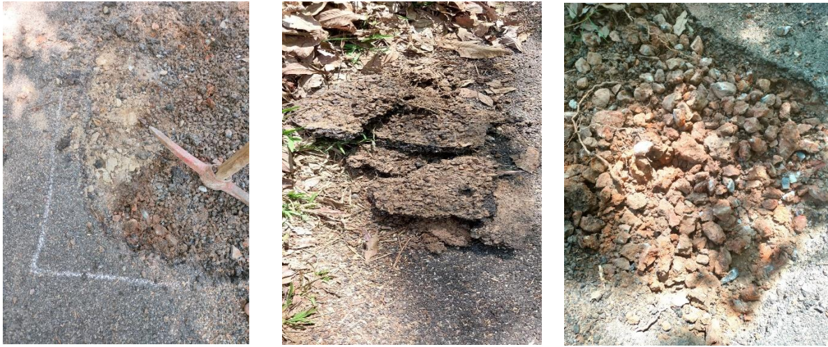
Fig 8: Separately collect various pavement layers
